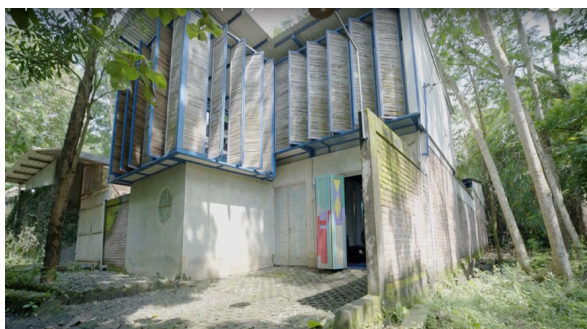
Figure 17. Front view of the building, illustrating
